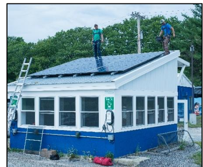
Image 8 - Solar panel installation for electric vehicle charging station on Portland Campus
