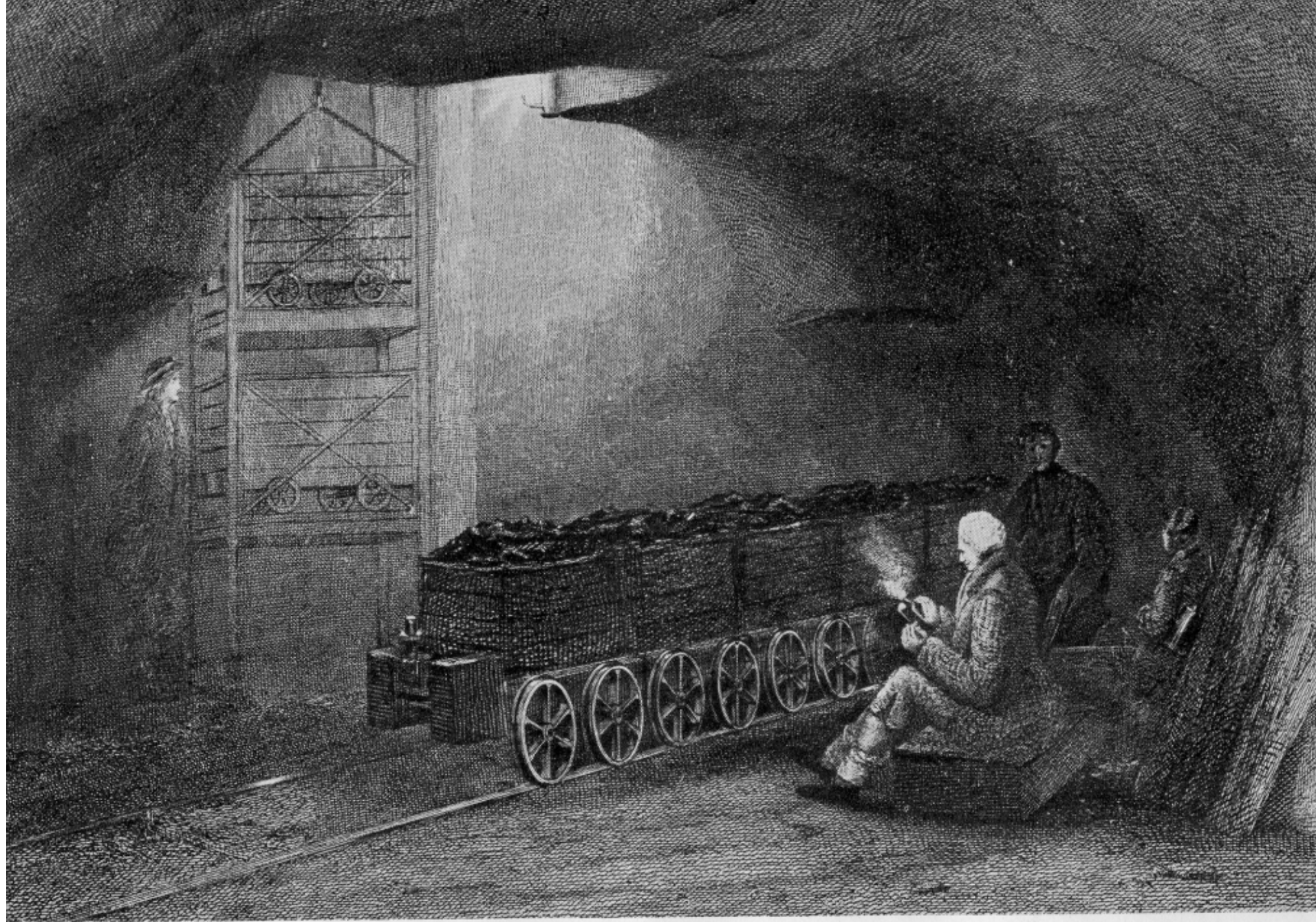
BOTTOM OF PIT SHAFT, 1860
